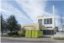
(a) Combined heat and power plant
